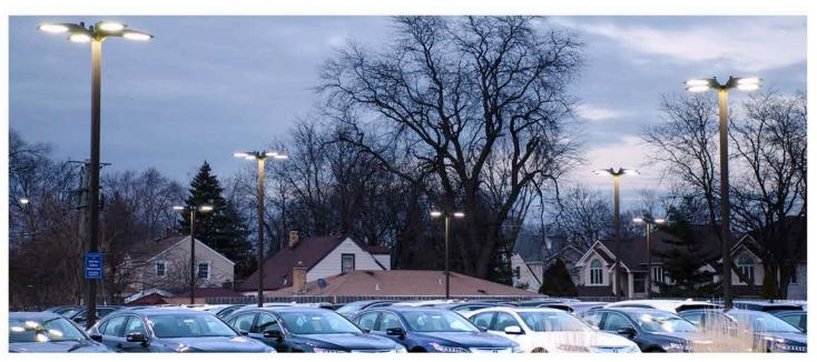
Summary - VLX fixtures - Replaced 72 fixtures Replaced 1000W pulse start with 359W LED fixtures
